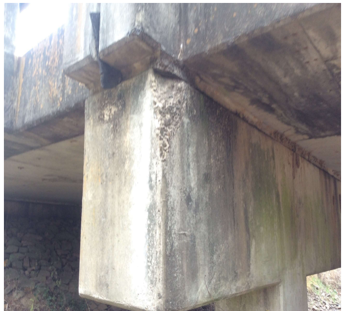
PHOTO 2 Description There is a 12" spall with no exposed reinforcing steel at the Rt side of Bent 2 cap.
