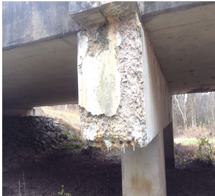
PHOTO 3 Description The Lt side of Bent 3 has soft deteriorated concrete with up to 4" of concrete section loss at this inspection. The ends of two reinforcement bars are visible at the base of cap. No apparent significant section loss to the exposed reinforcing steel.
