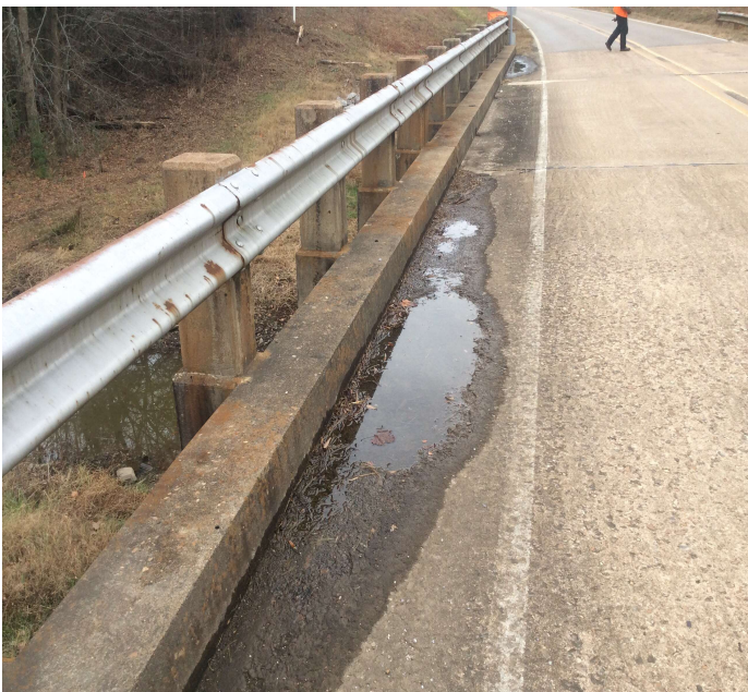
PHOTO 1 Description The left gutter has areas with heavy scale.
