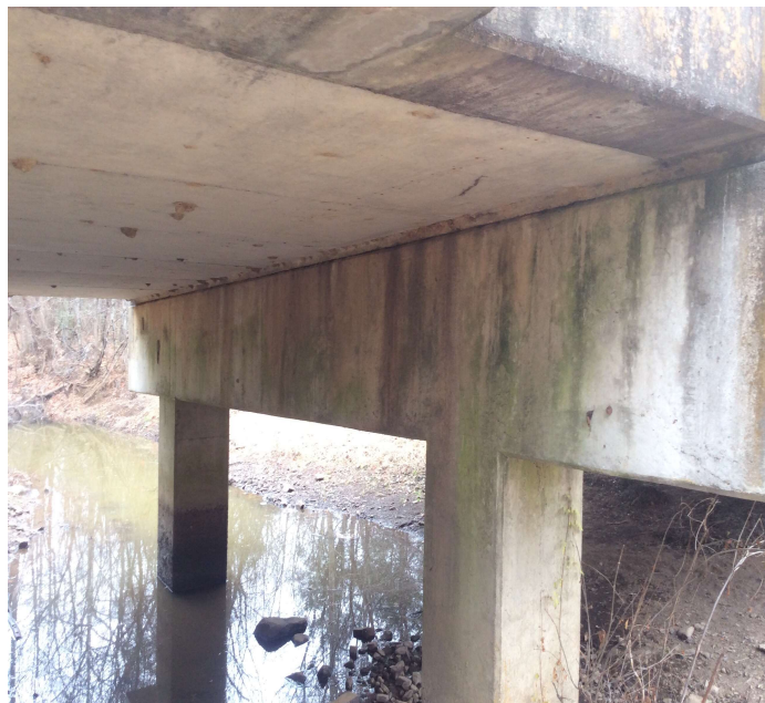
PHOTO 1 Description Substructure caps have efflorescence and water stains that appear to be an indication of leaking expansion joint sealant.
