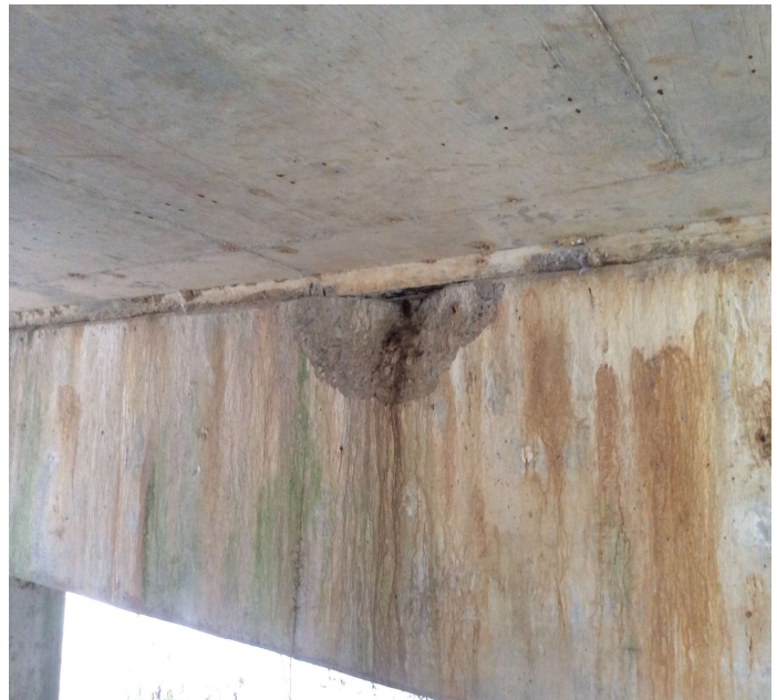
PHOTO 4 Description The Span 3 side of Bent 3 cap has a 24" spall with exposed reinforcing steel near the centerline of cap. No apparent section loss to the exposed reinforcing steel.
